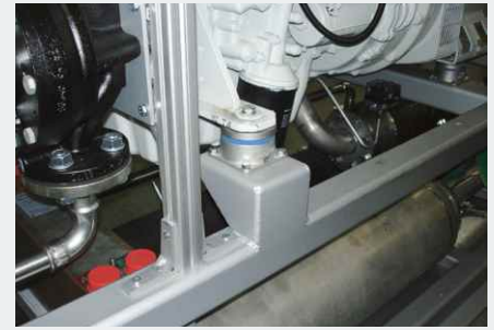
Pump with Isotop® DZE to compensate for high dynamic operating forces
