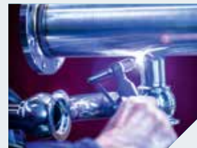
Orbital welding of a pigging station
