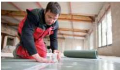
**Test assembly**: 80 mm cement screed (179 kg/m²) 16 mm AFM 33
