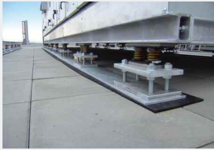
On-roof installation of an AC system with relatively high wind loads
