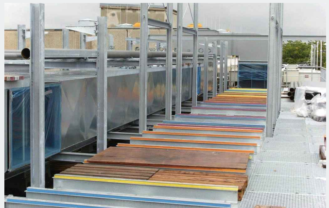
Strip bearing positioned in readiness for a rooftop ventilation unit
