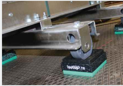
Vibration decoupled bearing of a distribution transformer
