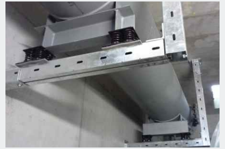
Bearing of duct silencer
