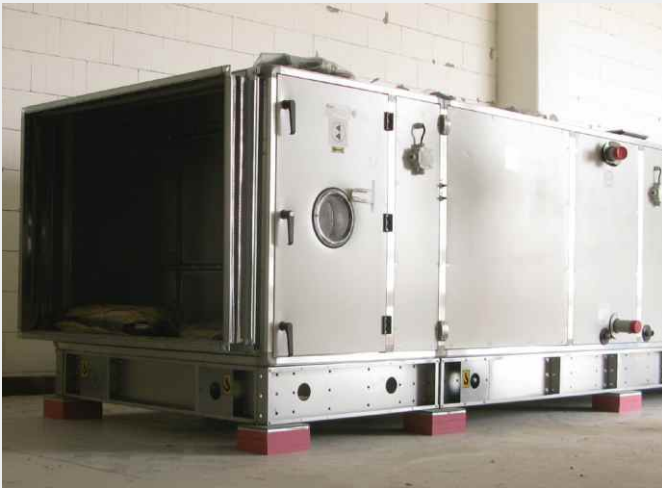
Bearing of an AC unit in the building
