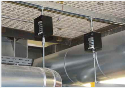
Decoupled pipes with SD/Z
