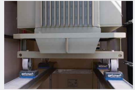
Vibration decoupled bearing of a distribution transformer
