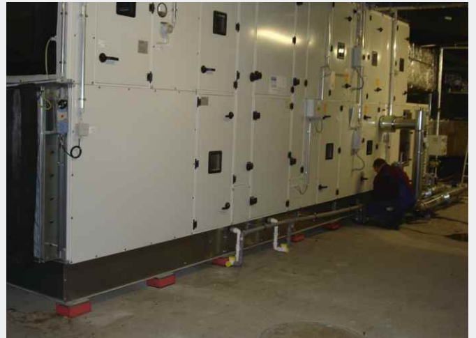
Installation of AC unit on Isotop® SE
