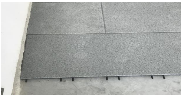
Each row should be offset by a half tile; tiles can also be cut around curves
