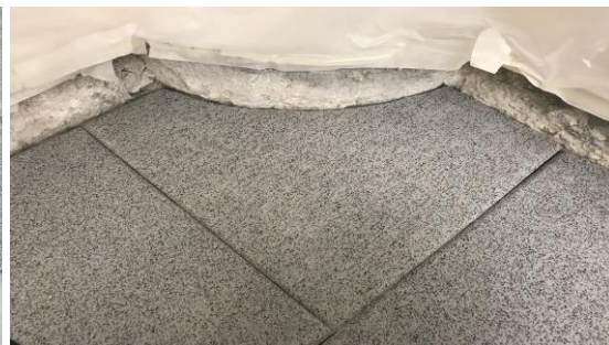
Each row should be offset by a half tile; tiles can also be cut around curves
