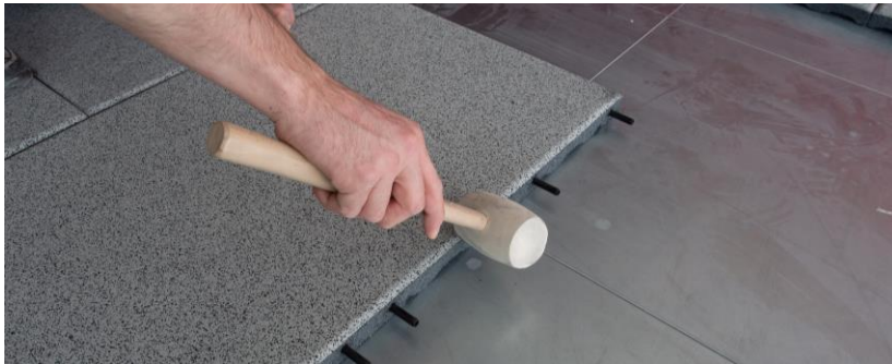
Closing the gaps with a hammer
