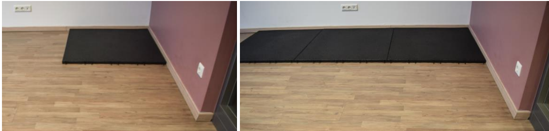
Installation of the tiles along a wall with the connector pins towards the next row
